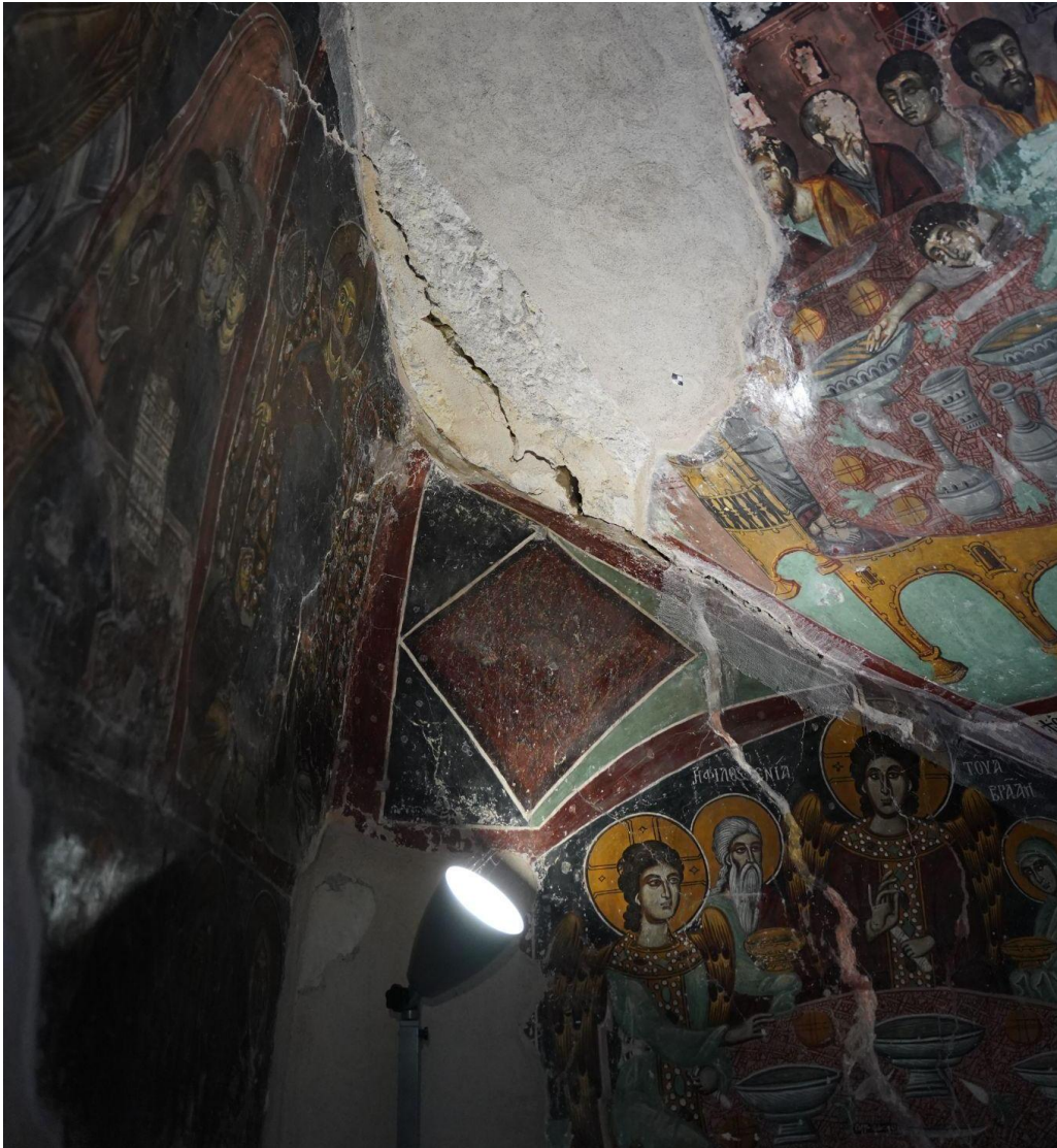
Figure 12: Photograph detailing previous conservation work.
